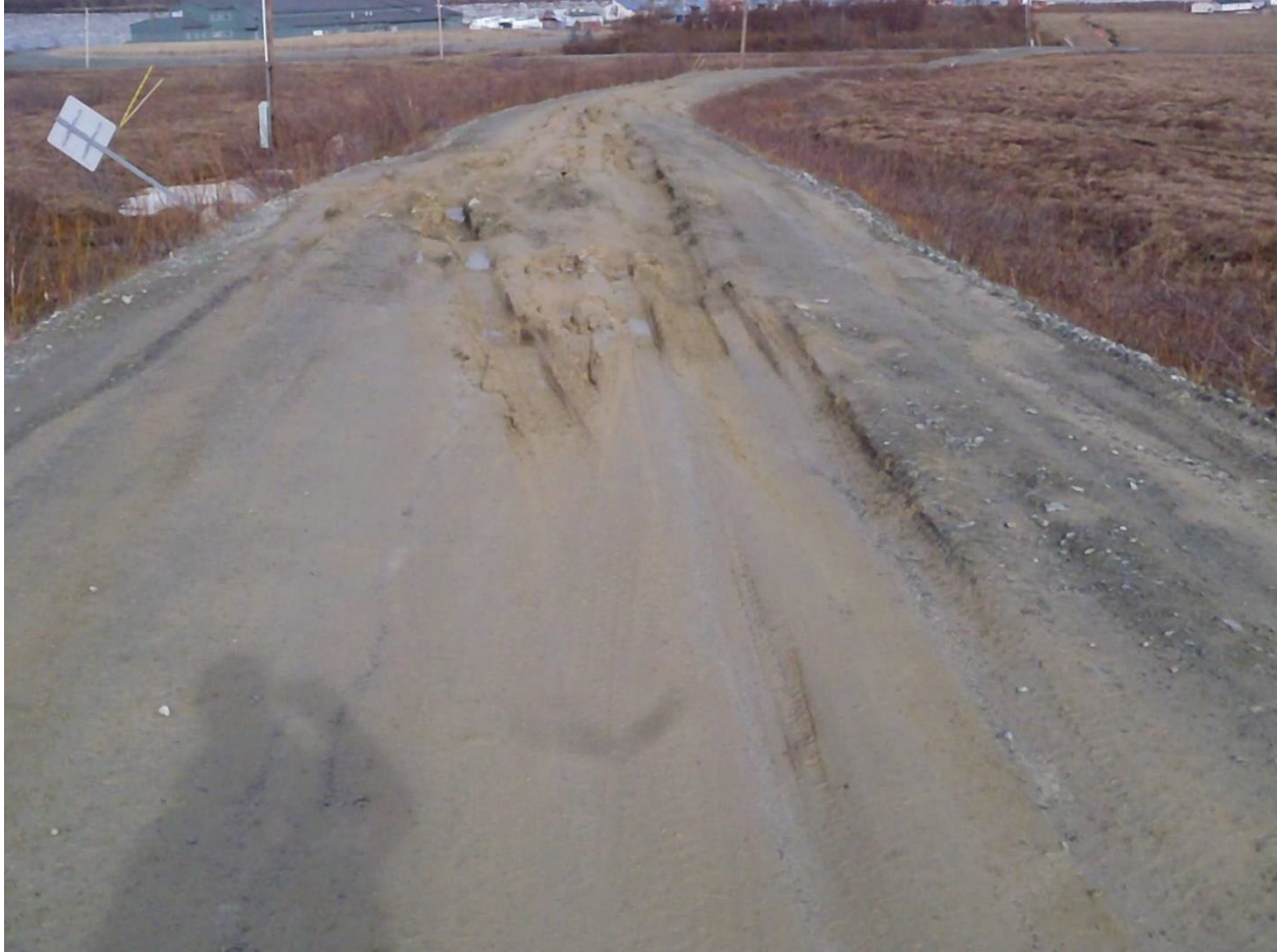
Graphic 3: Current Access Road (2022 AKDOT&PF photo taken by Chris Johnston)
