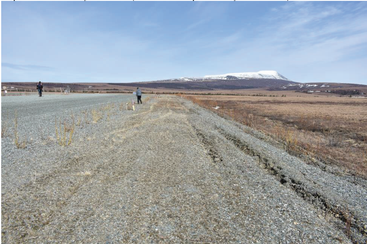
Graphic 1: Current Taxiway Embankment (2022 AKDOT&PF photo taken by Chris Johnston )
