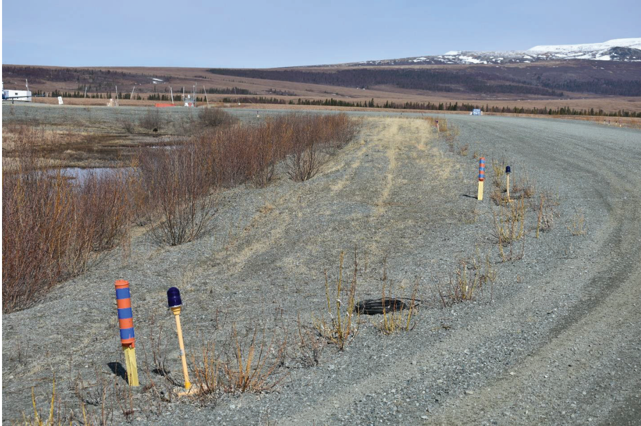
Graphic 2: Current lighting (2022 AKDOT&PF photo taken by Chris Johnston)
