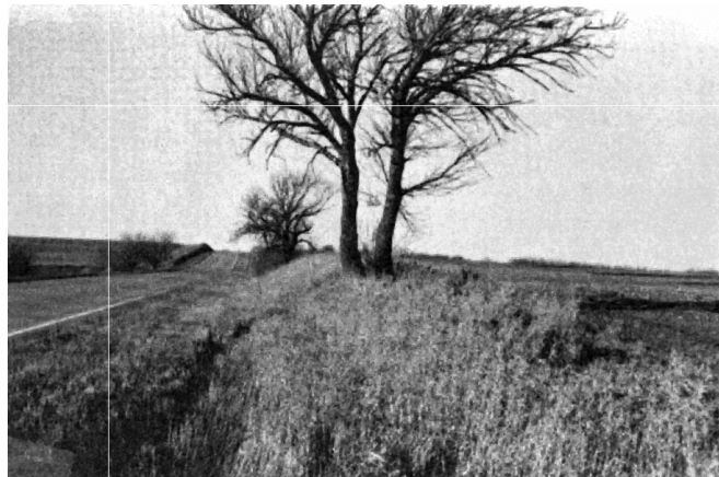
Figure 1160-4 Rural Roadside Hazard Rating of 4
